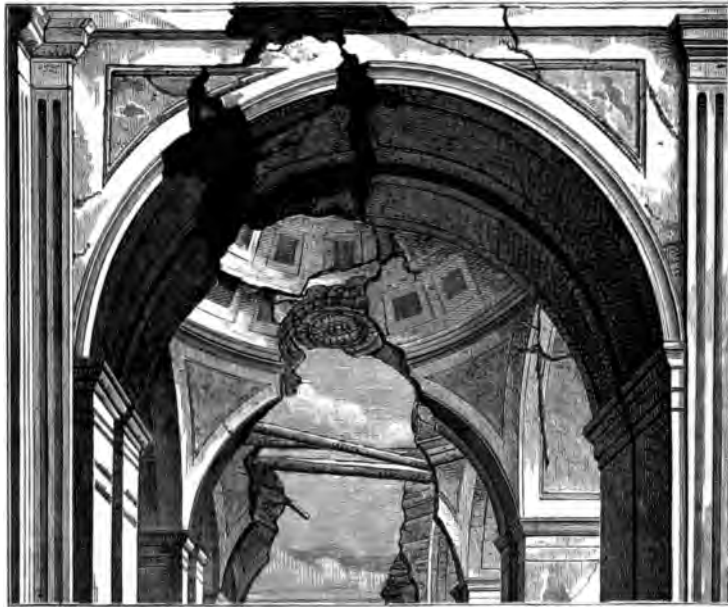
FIG. 112.—CATHEDRAL OF TITO, CALABRIA, AFTER THE EARTHQUAKE OF 1857. (After Mallet.)
